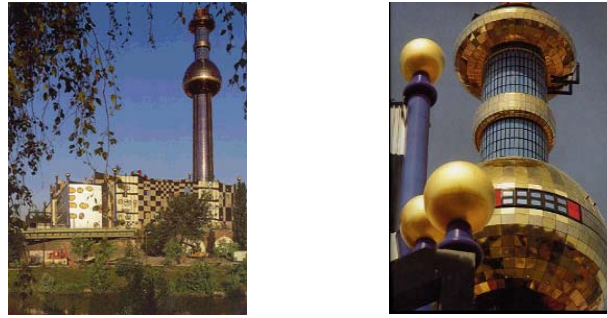
Figure 7: Vienna's Waste to Energy CHP Plant
