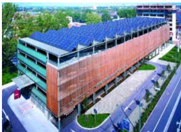
Figure 2: Multi-storey car park 3
